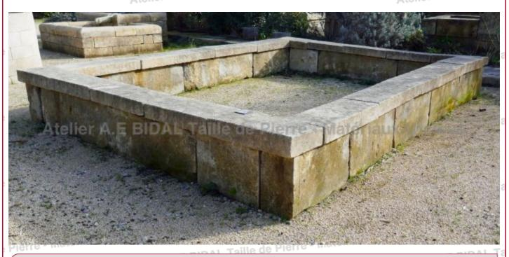
Large ancient basin made of reclaimed stones. Basin or rectangular shape. This basin has wide and thick copings. It is made of natural stone from South of Provence called "buget".
